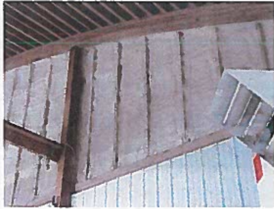
Spray insulation has been added to portions of the interior walls.
