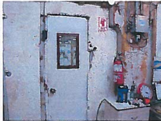
Spray insulation has been added to portions of the interior walls.
