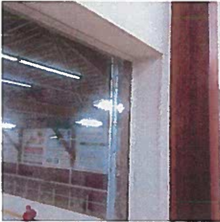
The community room has a removable window to allow for the transfer of chairs and tables down to the rink floor for certain community events.
