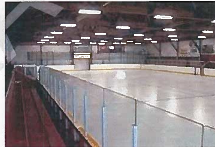
Existing Ice Pad at NDCC
