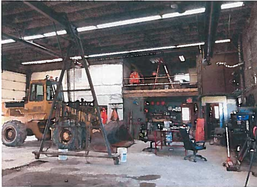
Photo 11: View of Second Floor Open Mezzanine and Slender Wood Guard Rail
