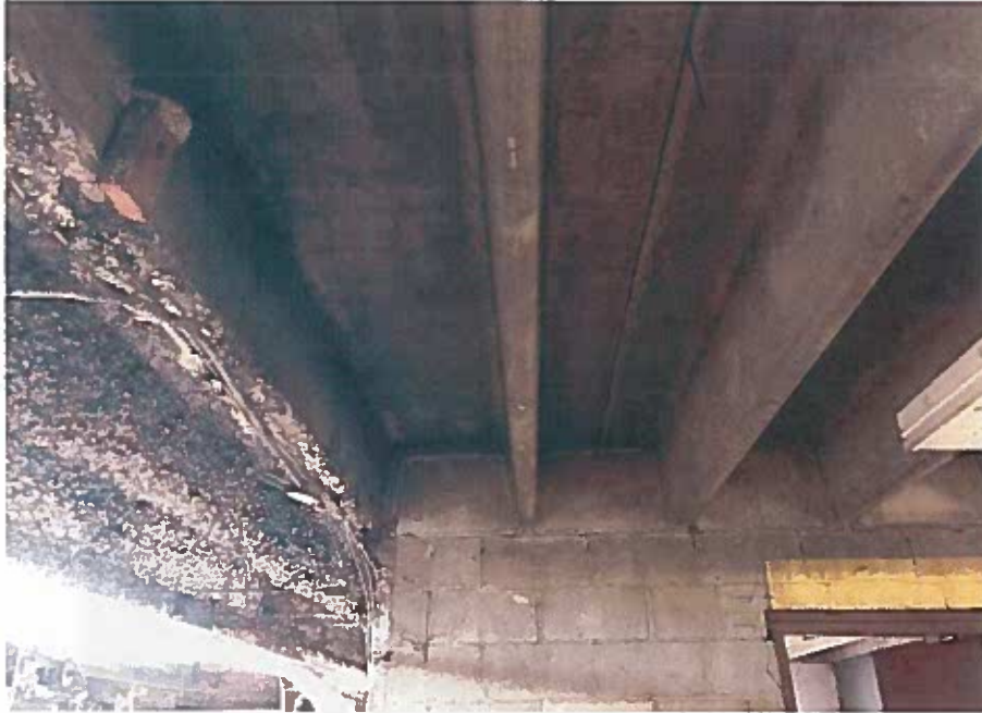
Photo 7: View of Precast Concrete Double Tees Above the Second Floor Area
