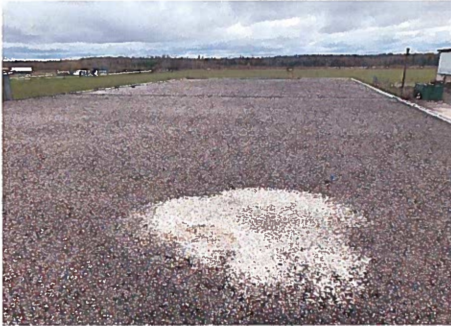
Photo 17: Overview of Roof Looking East
