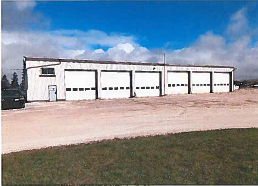
Photo 1: South Elevation, Office on West End, Newer Addition on East End
