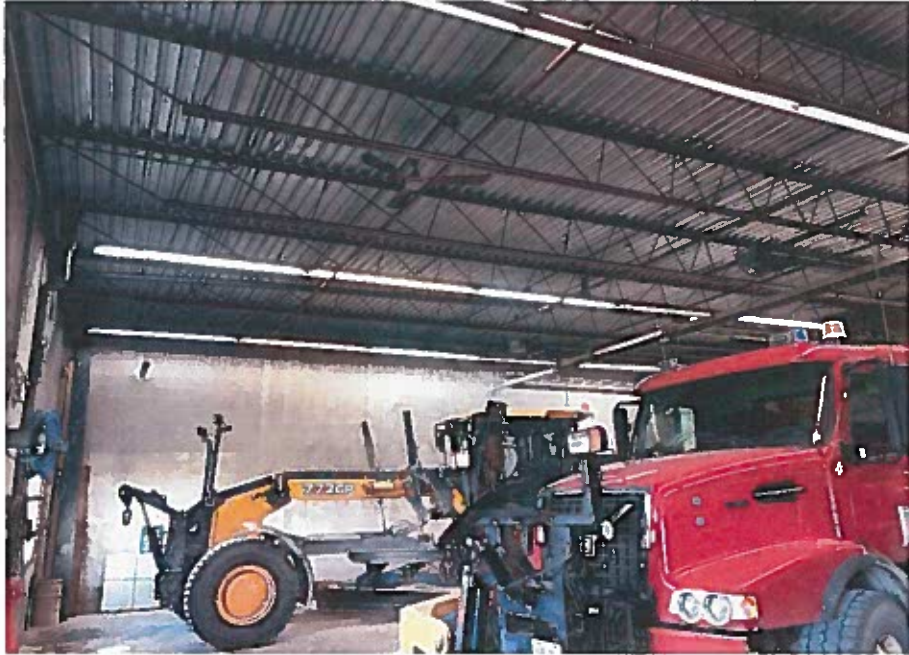
Photo 15: View Inside Garage Addition Showing Open Web Steel Joist Roof Structure
