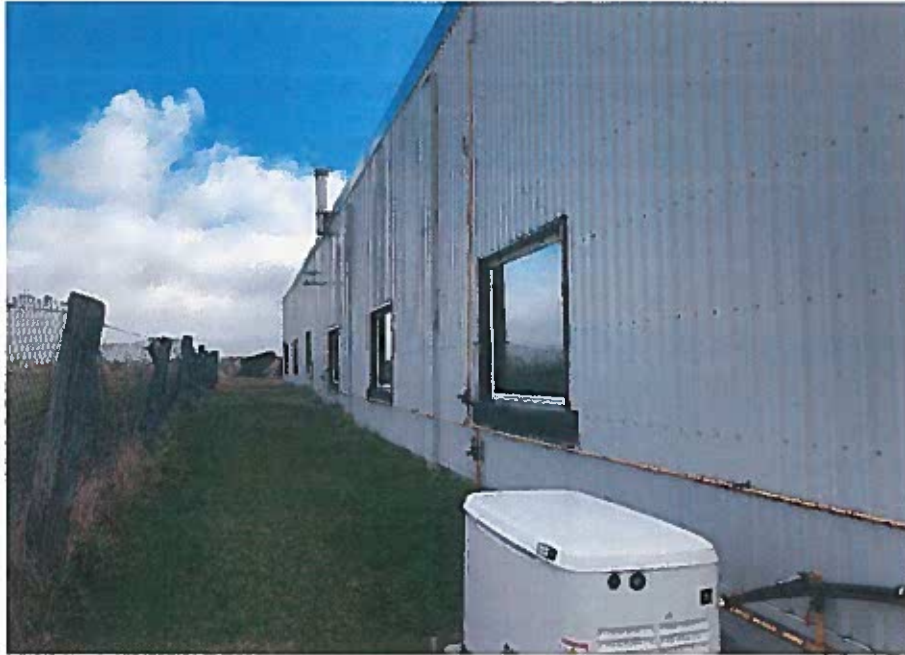
Photo 3: North Elevation Viewed from West Side
