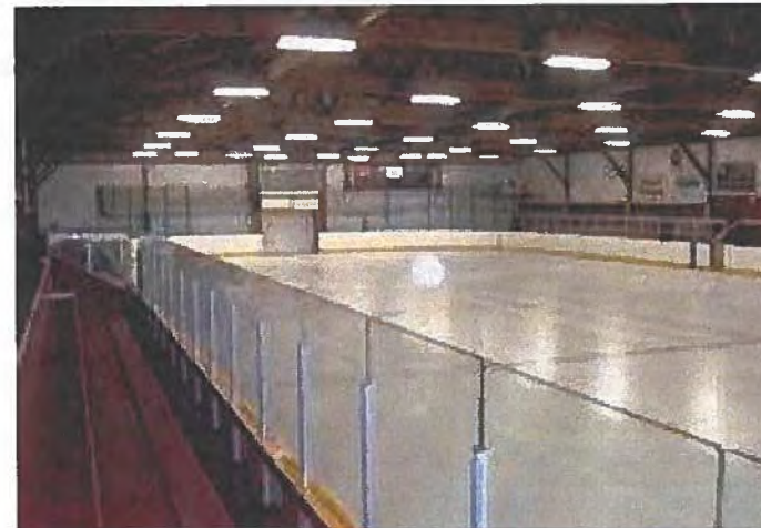
Existing Ice Pad at NDCC
