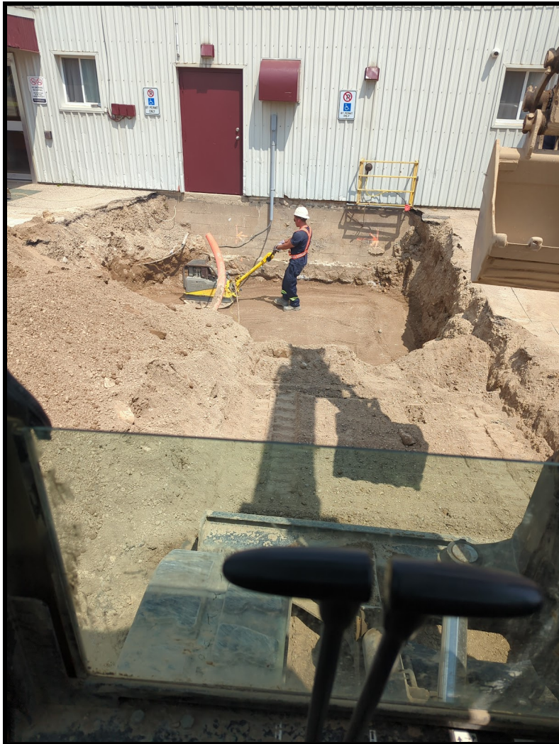
Figure 4: Compacting Backfill Material. Facing East.
