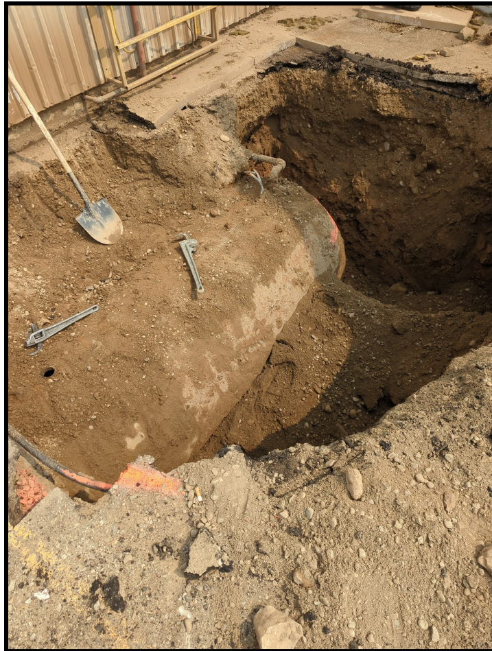
Figure 3: Underground Storage Tank Location. Facing Southeast.
