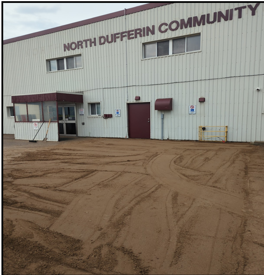
Figure 5: Backfilled Area. Facing Northeast.
