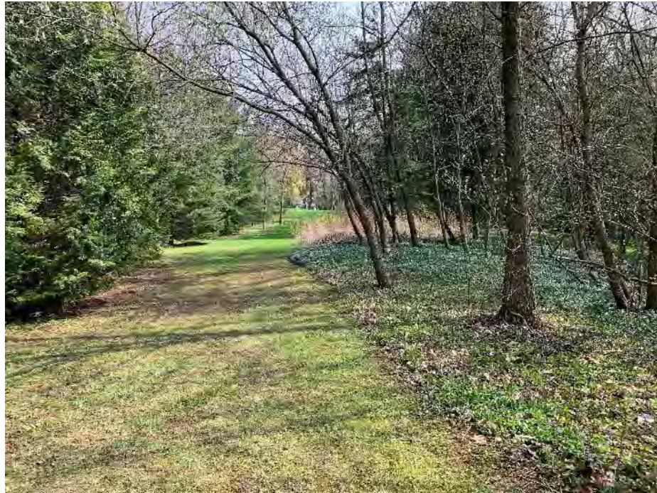
Photograph 15: Alternate view of toe area of slope
