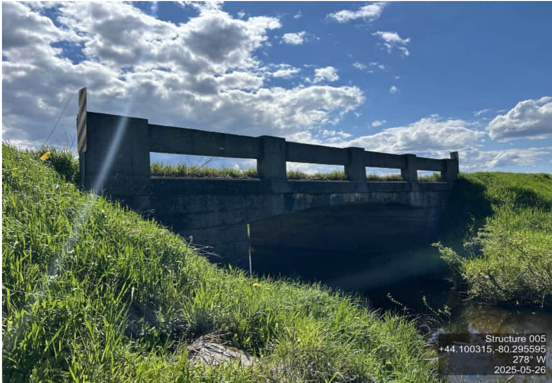
STREAM – THROUGH STRUCTURE – STREAM FLOWS ON A SKEW
