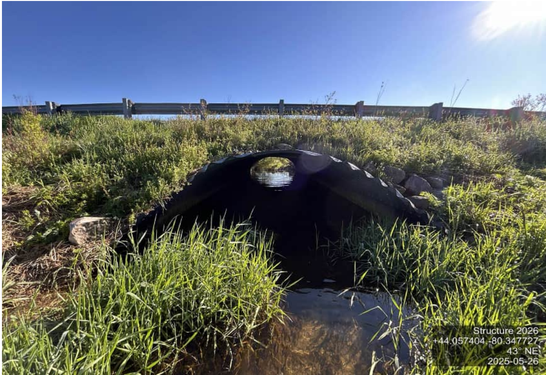
ELEVATION SHOT – NORTHEAST
