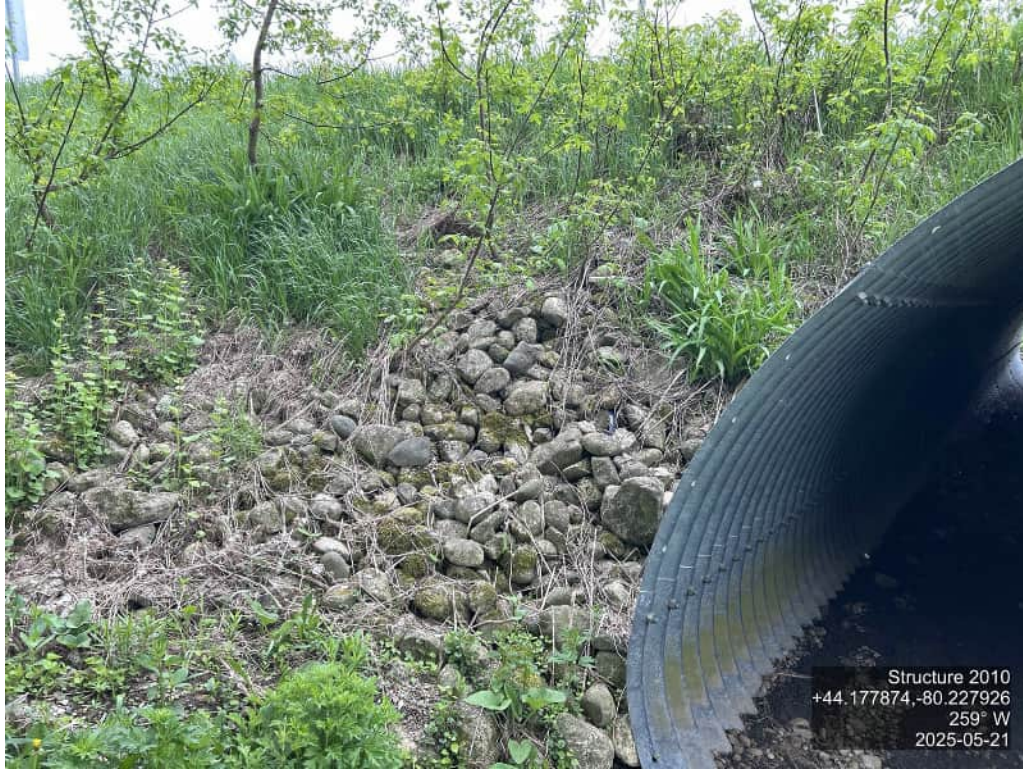
EMBANKMENT – EAST – SLOPE PROTECTION
