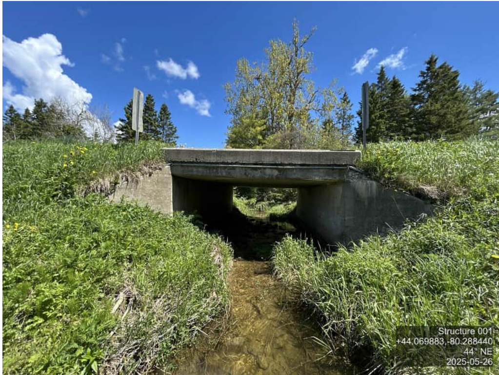
ELEVATION SHOT – NORTHWEST
