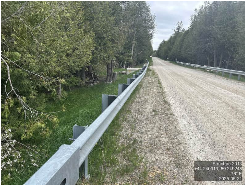
APPROACH WEARING SURFACE – EAST
