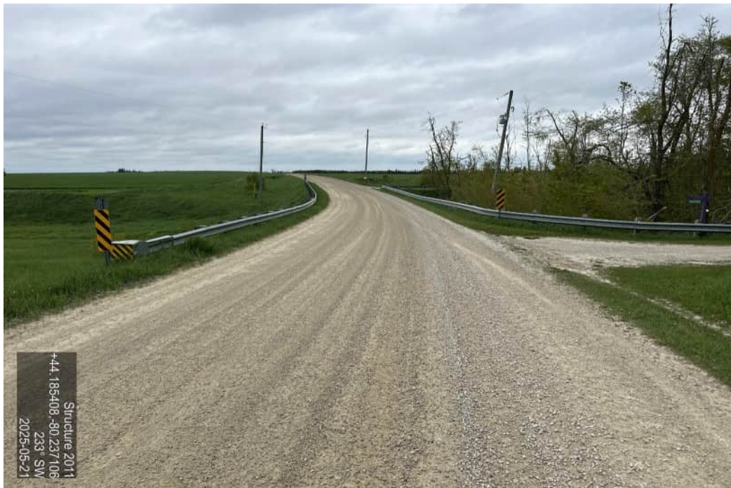
APPROACH WEARING SURFACE – EAST
