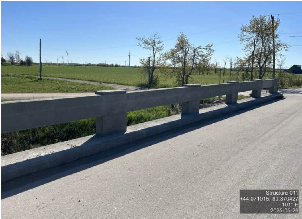
RAILING SYSTEM – SOUTH – REPAIRED DURING 2022 REHAB
