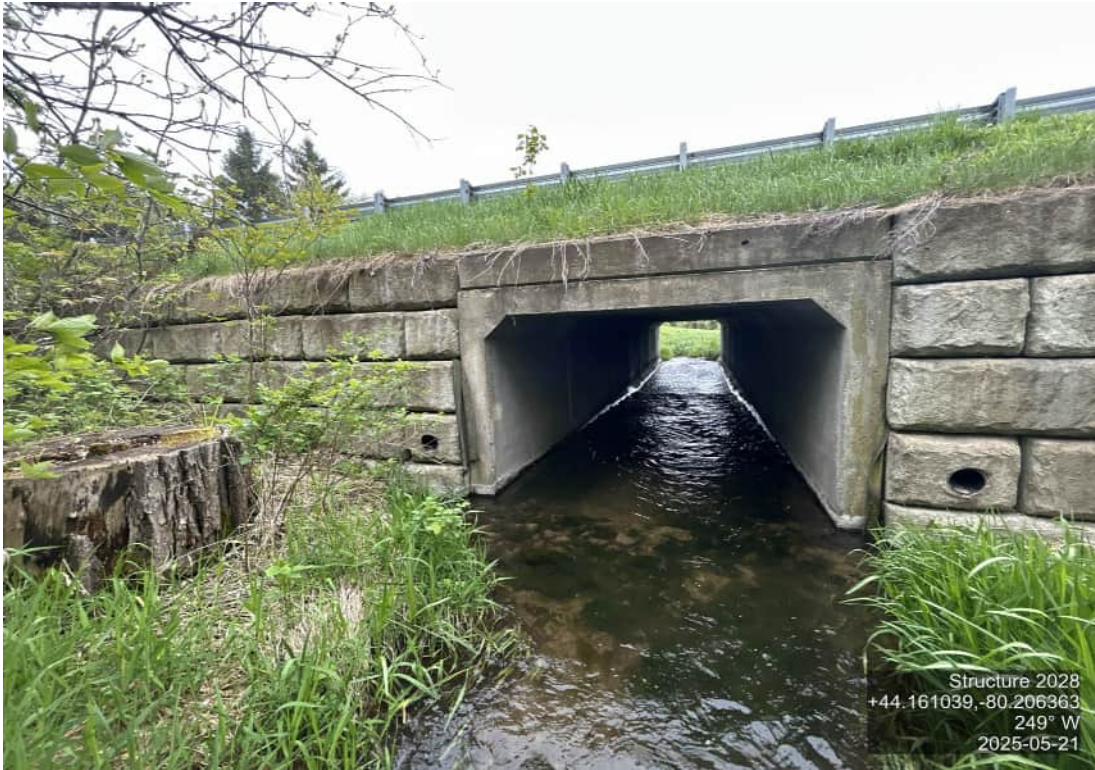
ELEVATION SHOT – EAST
