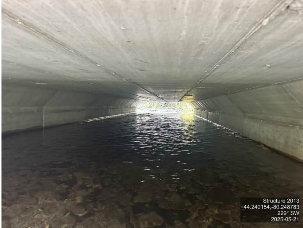
BARREL – CULVERT INTERIOR
