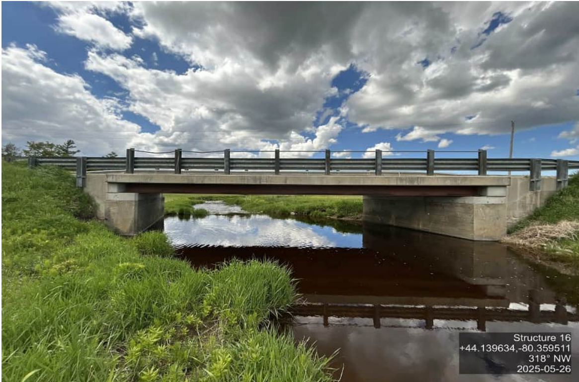
ELEVATION SHOT – WEST
