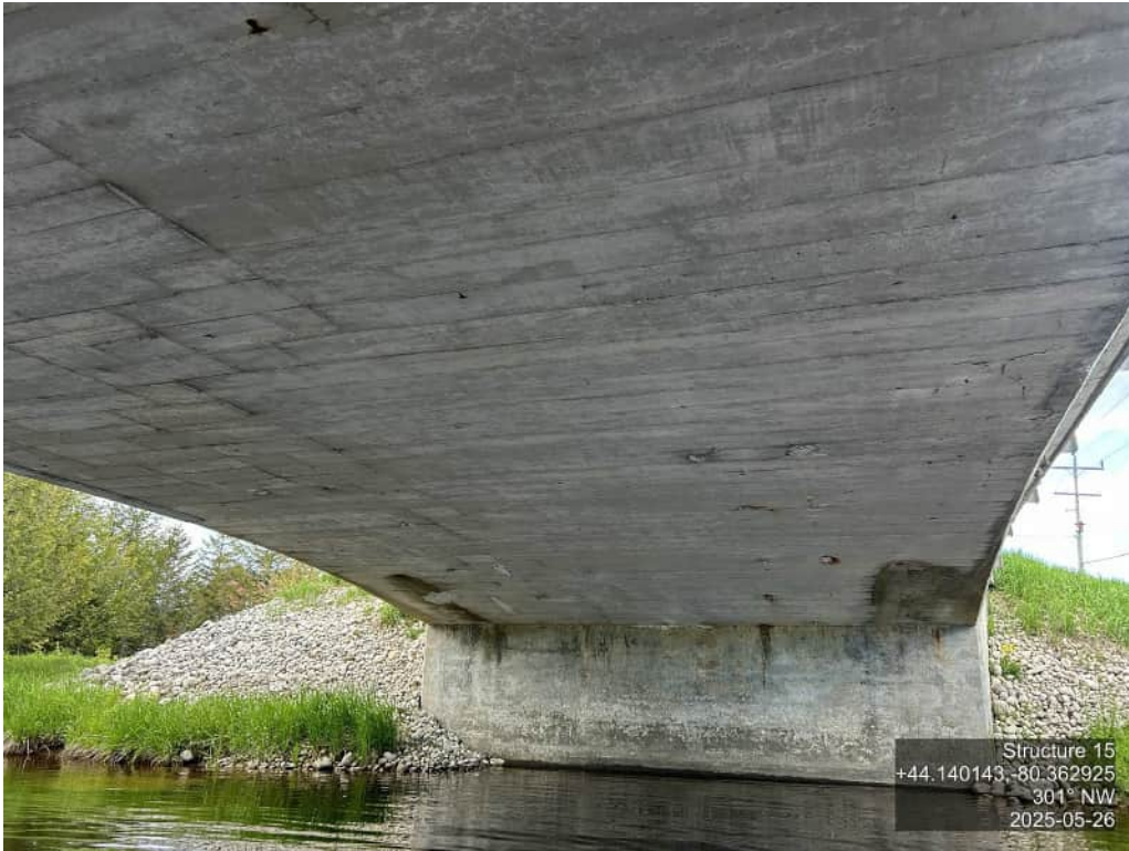
EMBANKMENT – ALL QUADRANTS – ROCK PROTECTION
