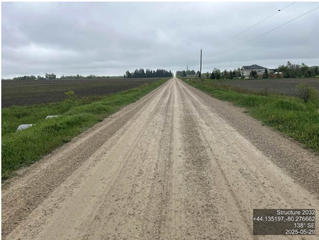
DECK WEARING SURFACE – SOUTH
