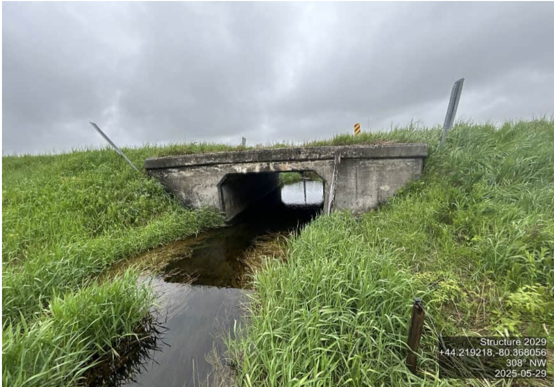
ELEVATION SHOT – WEST
