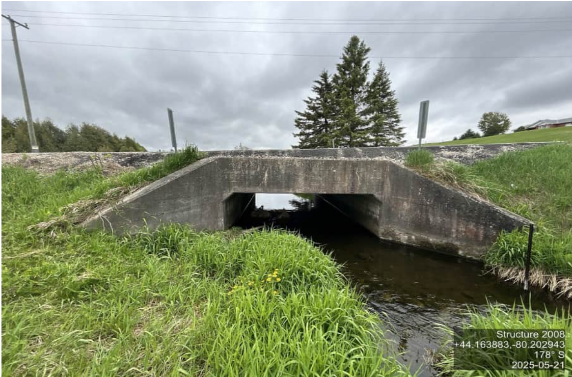
ELEVATION SHOT – LOCATION - DESCRIPTION
