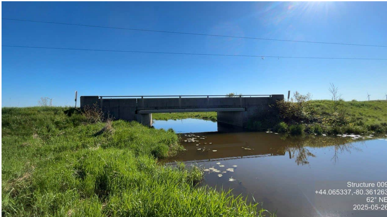
ELEVATION SHOT – NORTHWEST
