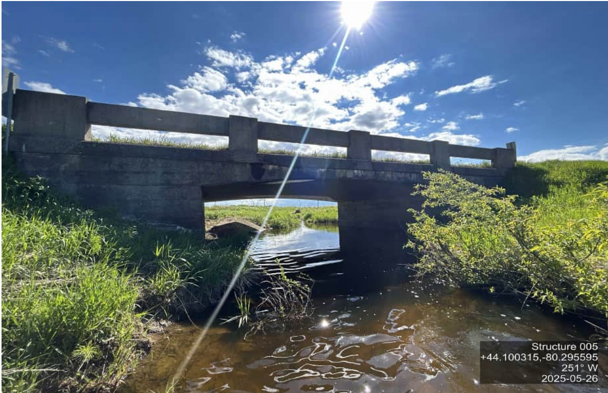
ELEVATION SHOT – WEST
