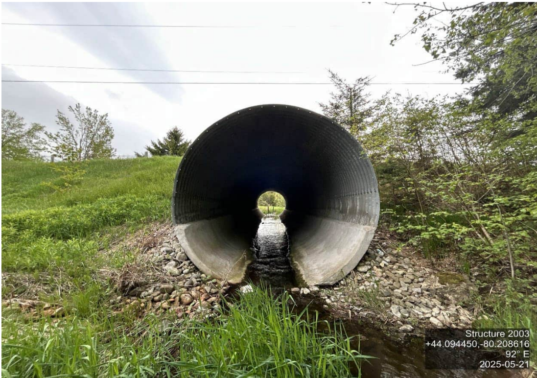
ELEVATION SHOT – WEST
