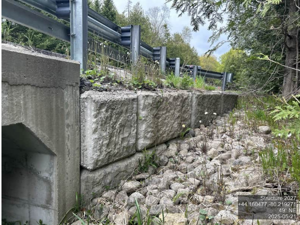
EMBANKMENT – SOUTHEAST – ROCK PROTECTION
