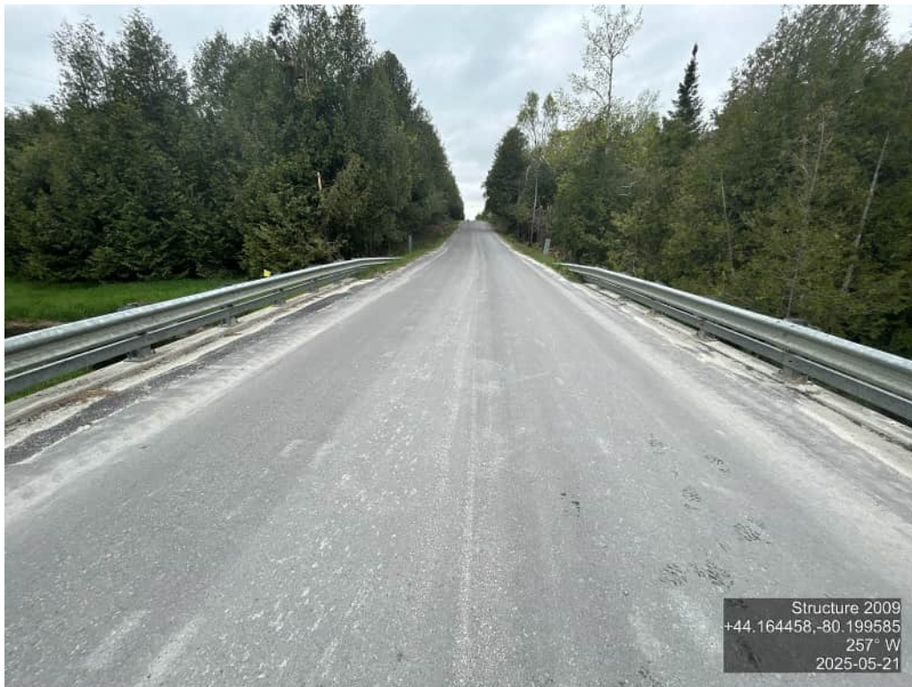
DECK WEARING SURFACE – WEST
