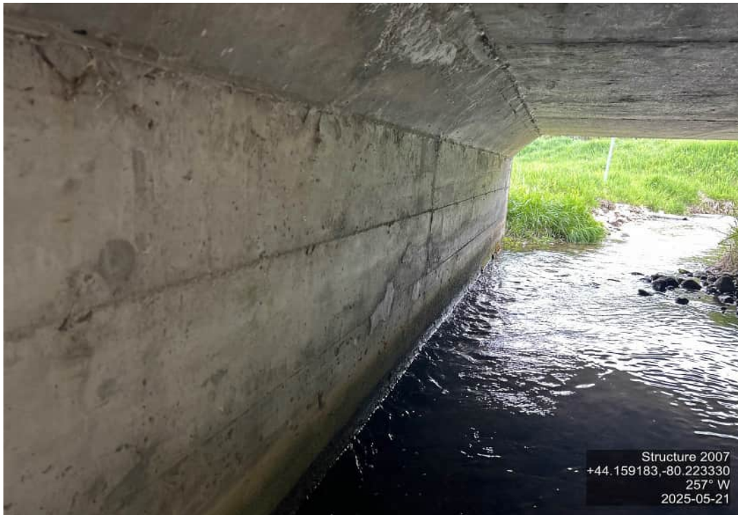
ABUTMENT WALLS – WEST
