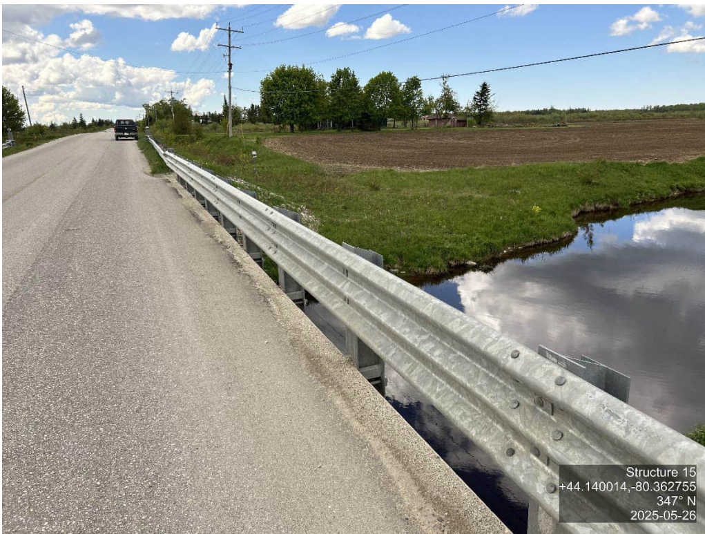
RAILING SYSTEM – WEST
