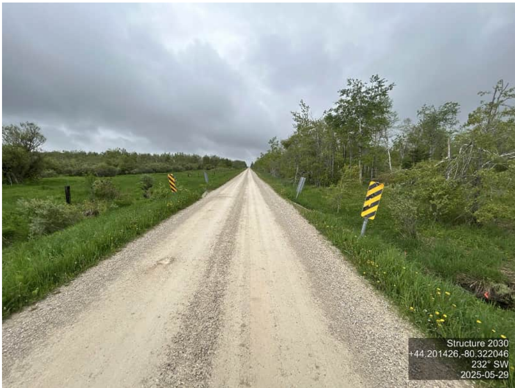
DECK WEARING SURFACE – SOUTHWEST – SMALL POTHoles
