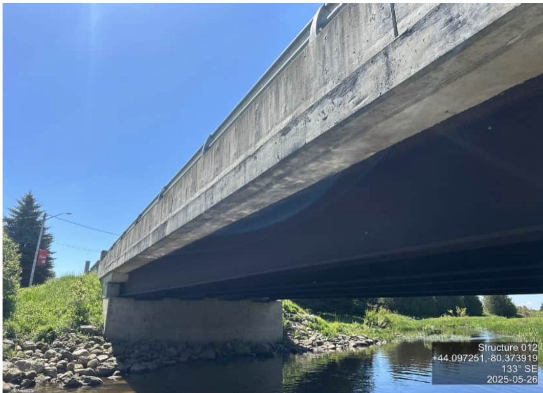
BARRIER WALLS EXTERIOR – SOUTHWEST
