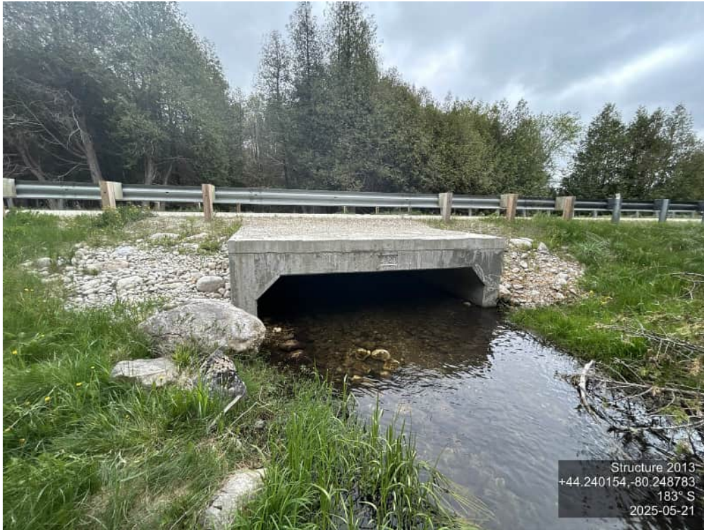
ELEVATION VIEW - NORTH
