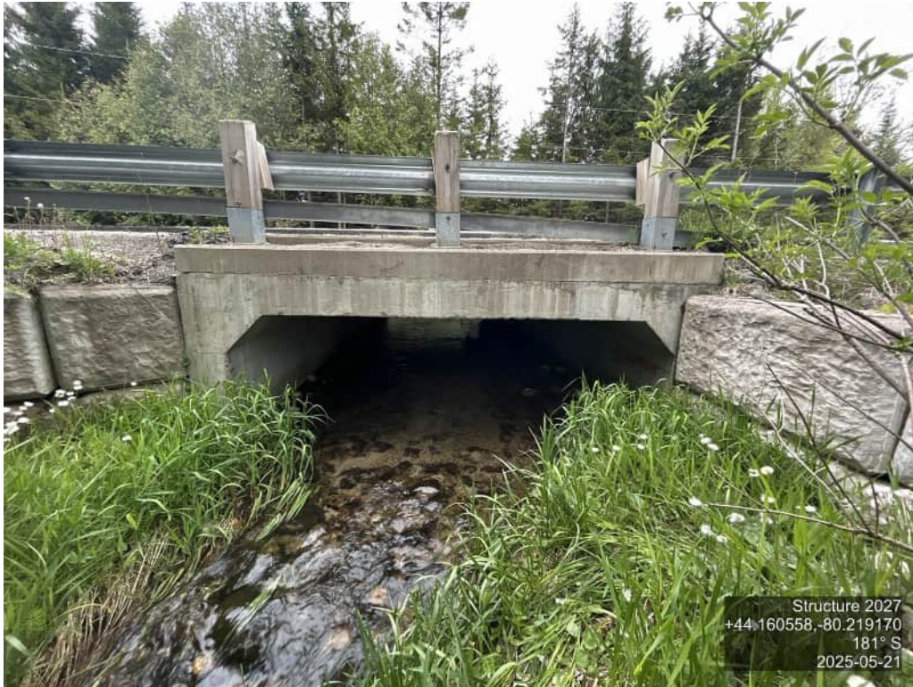
ELEVATION SHOT – SOUTH
