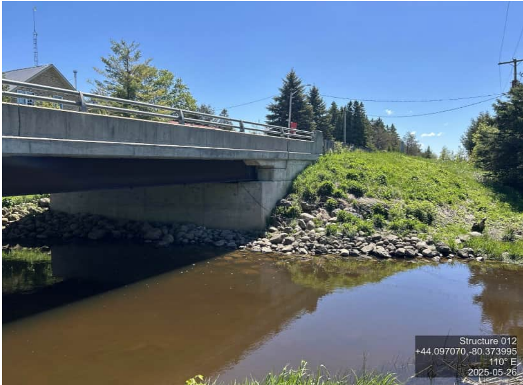
EMBANKMENTS – SOUTHEAST – ROCK PROTECTION
