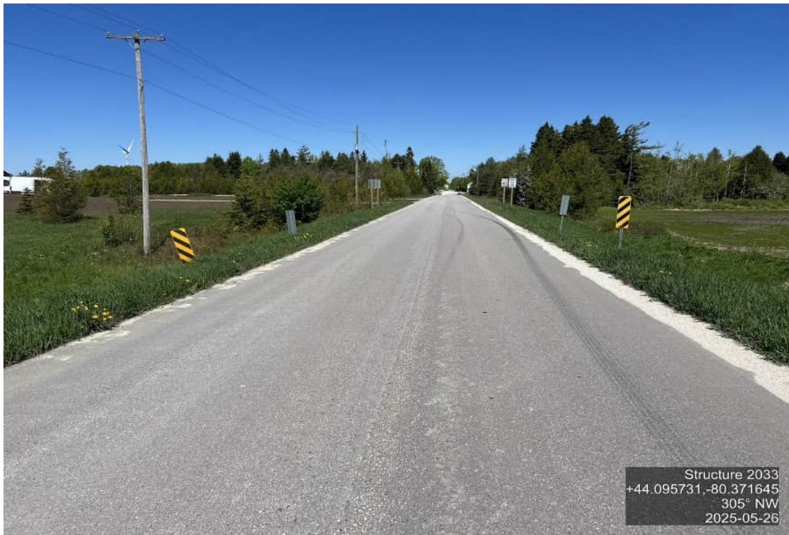
DECK WEARING SURFACE – NORTH – RE-PAVED IN 2023
