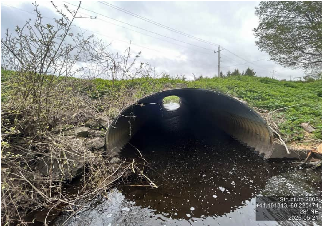
ELEVATION SHOT – NORTHWEST
