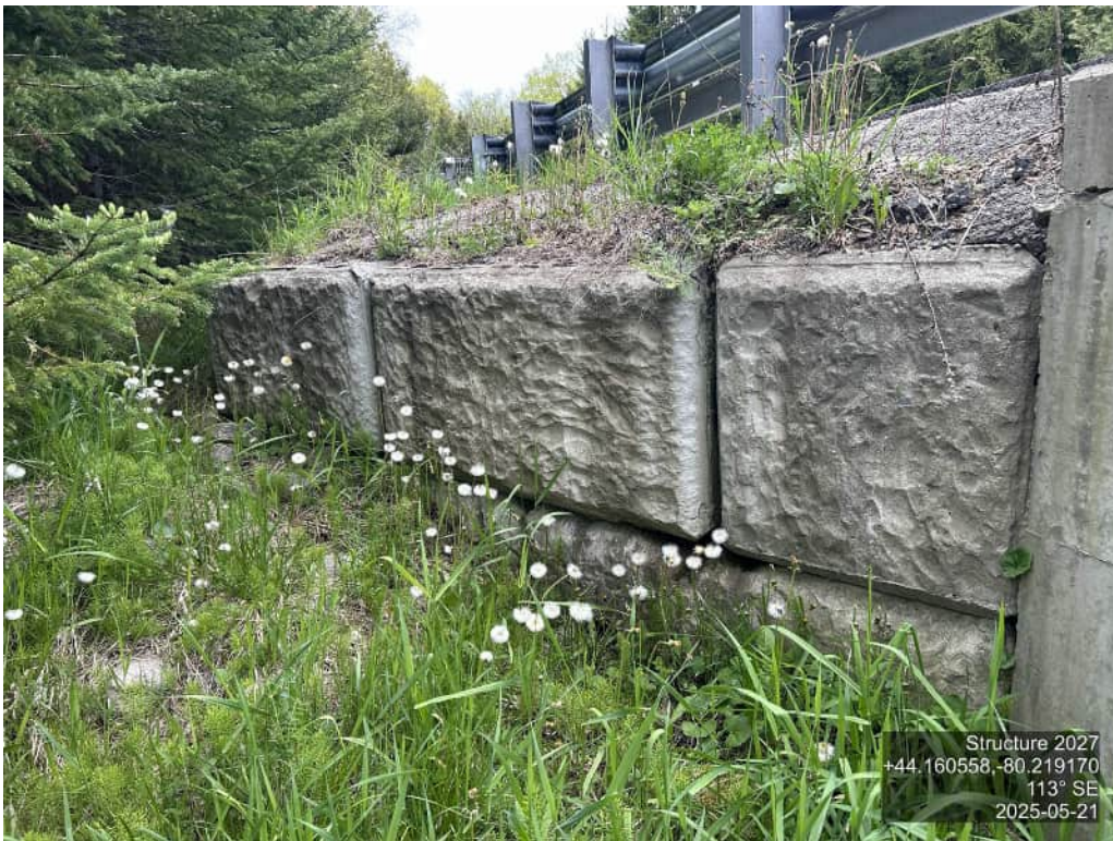
RETAINING WALL – SOUTHEAST
