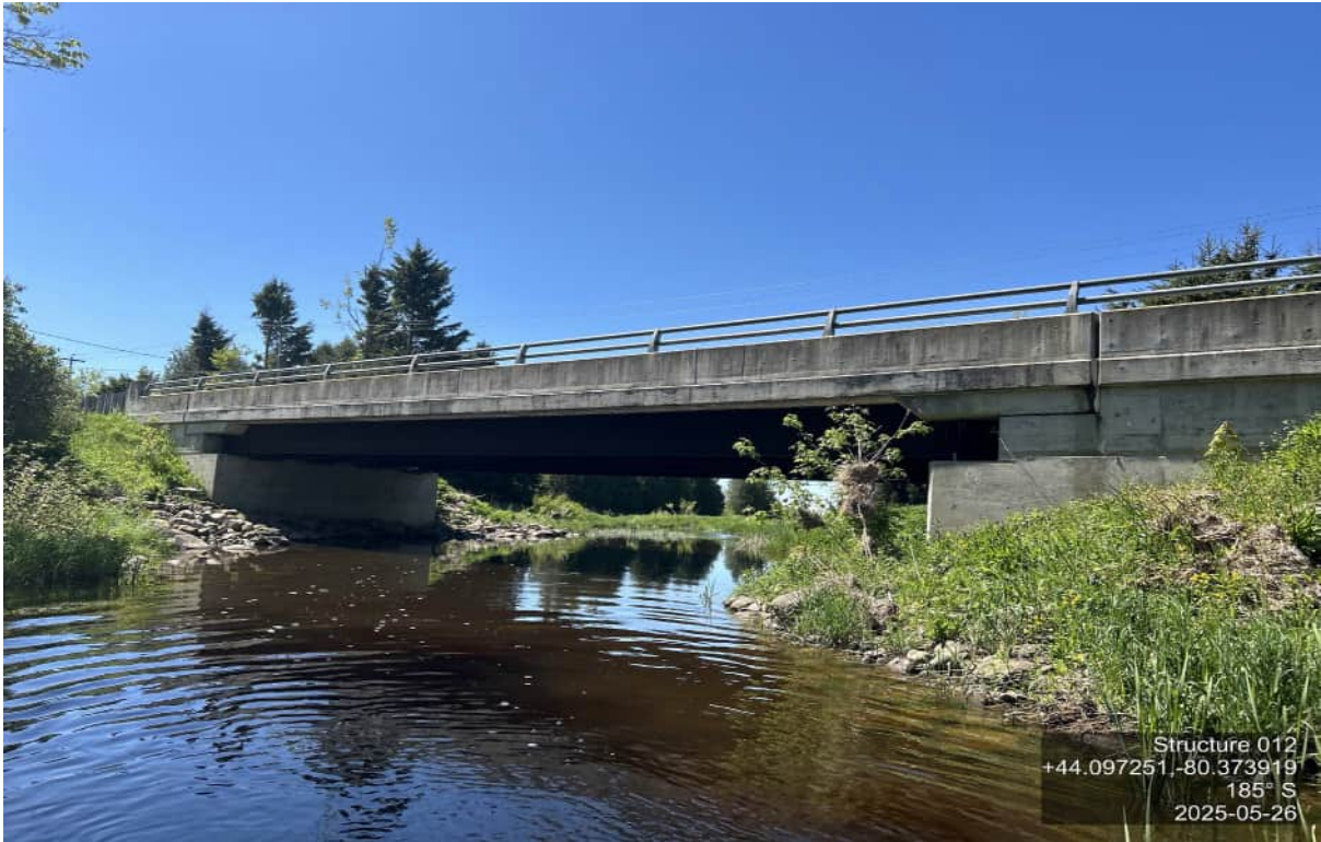
ELEVATION SHOT – NORTH
