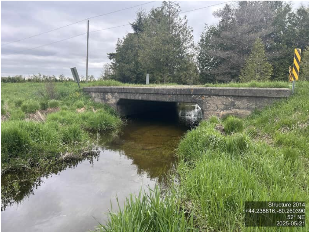
ELEVATION SHOT – EAST
