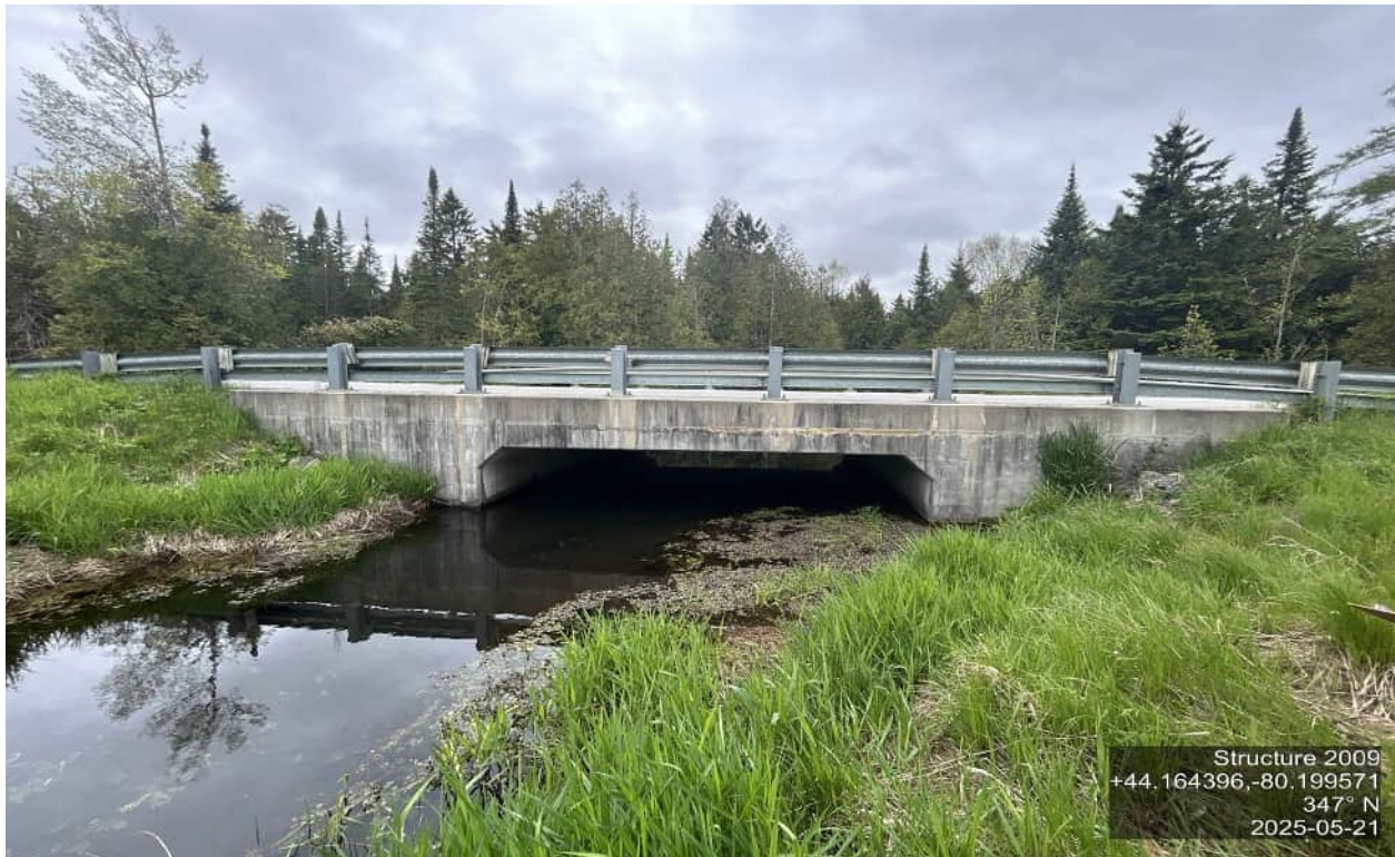
ELEVATION SHOT – NORTH
