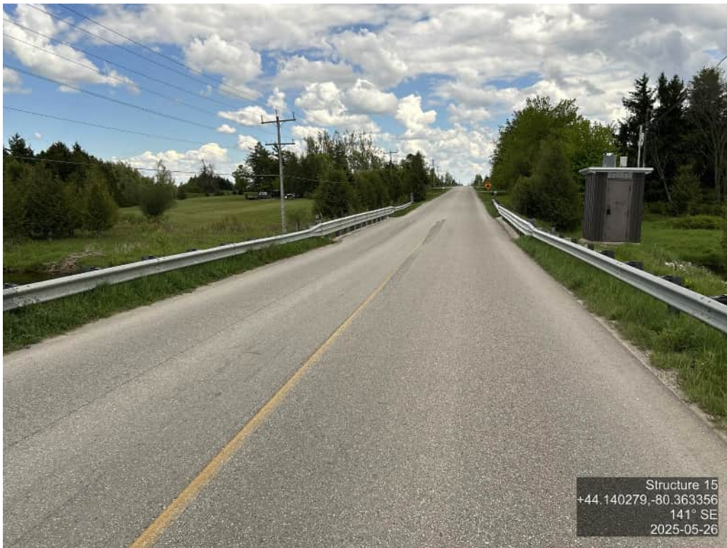
APPROACH WEARING SURFACE – SOUTH
