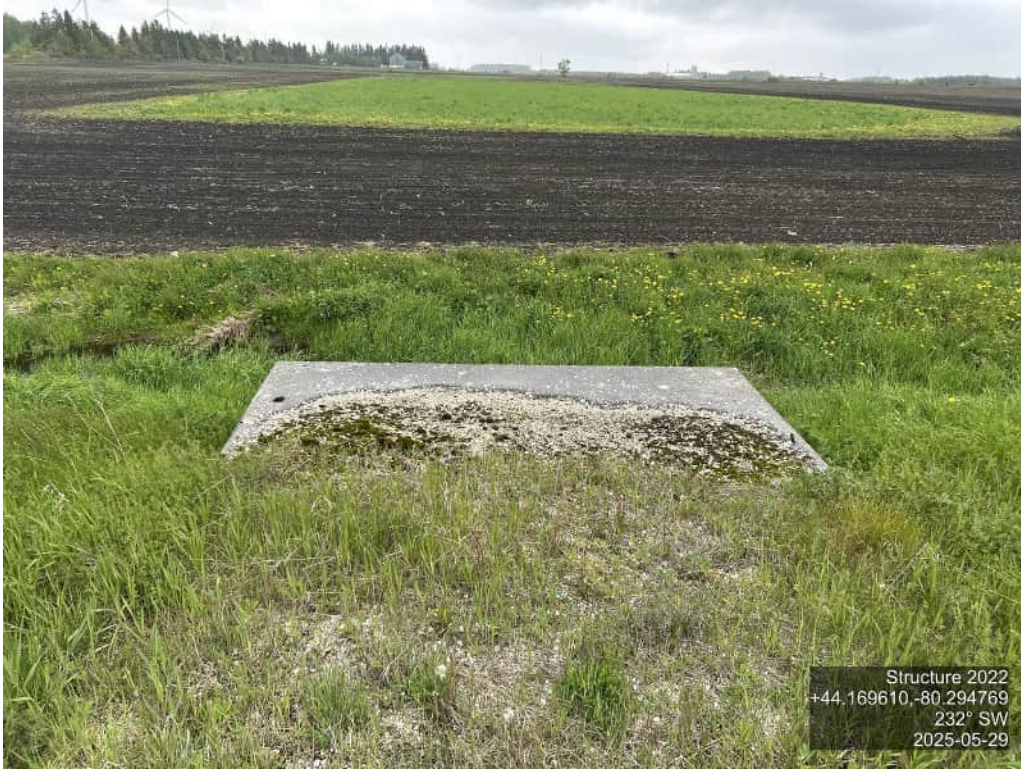
EMBANKMENT – NORTH – WELL VEGETATED
