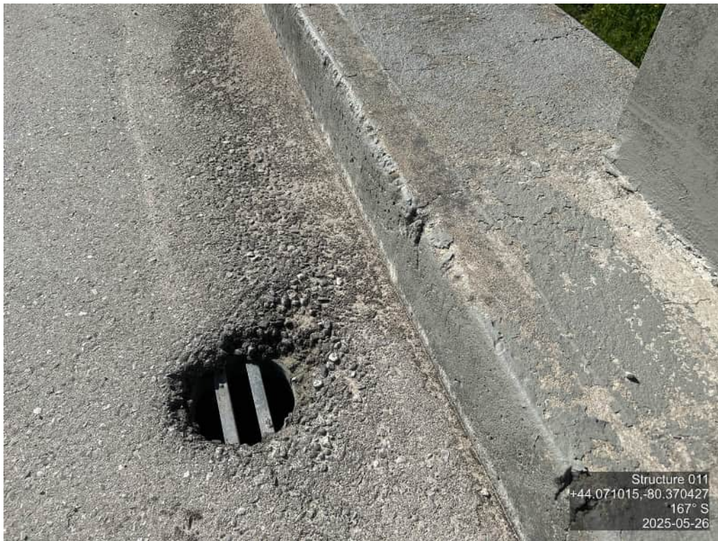
DECK DRAINS – EAST – ALL APPEAR FUNCTIONAL
