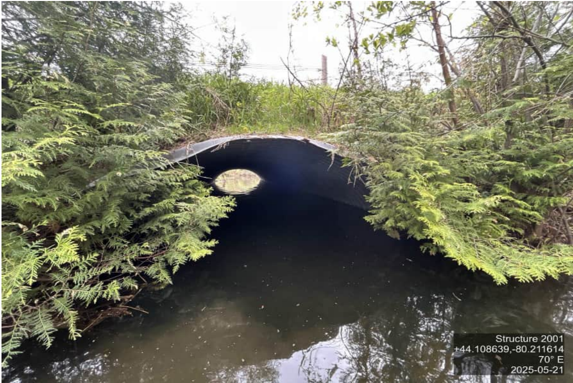
ELEVATION SHOT – EAST
