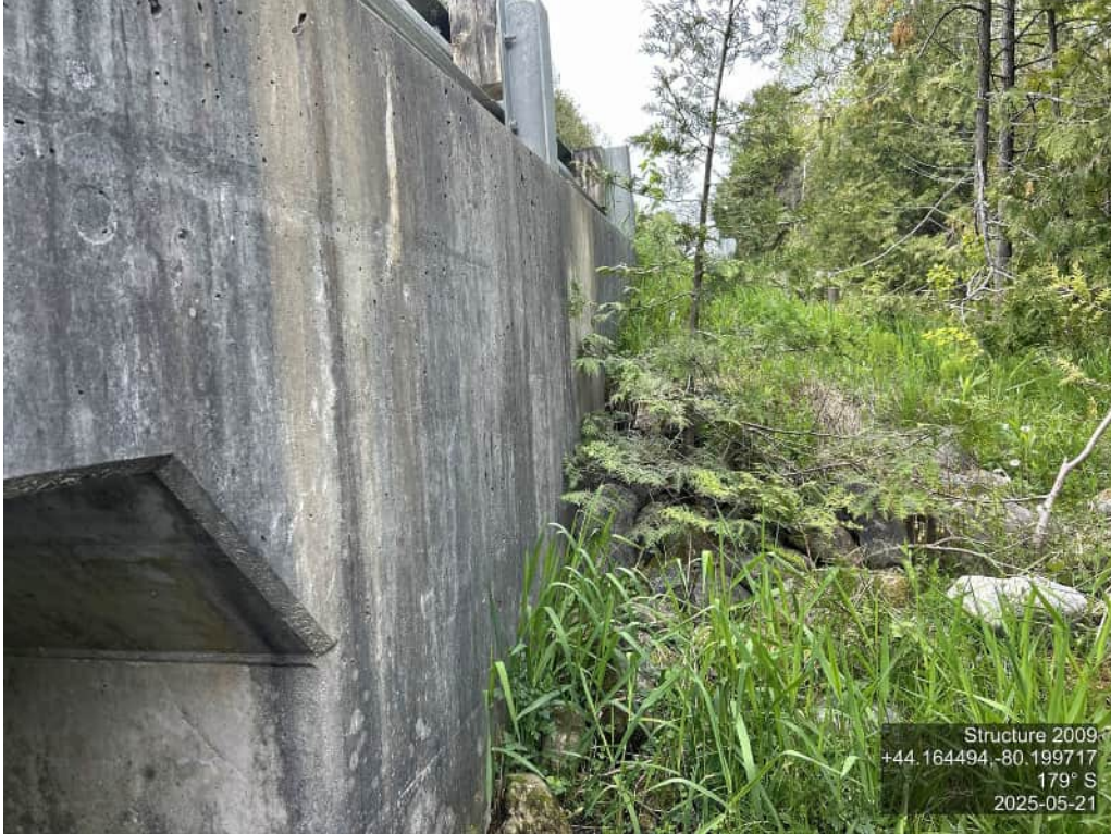
EMBANKMENT – NORTHEAST – ROCK PROTECTION
