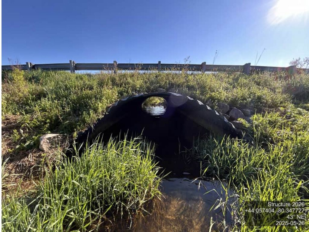
EMBANKMENT – NORTHEAST – STABLE WITH ROCK PROTECTION
