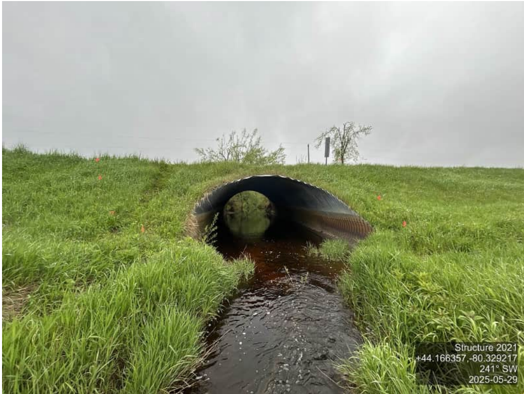
ELEVATION SHOT – WEST
