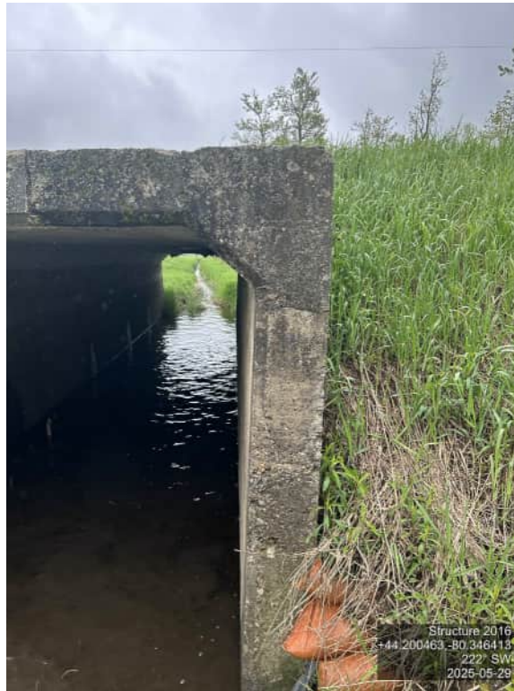
EMBANKMENT – SOUTHEAST – SANDBAGS PRESENT
