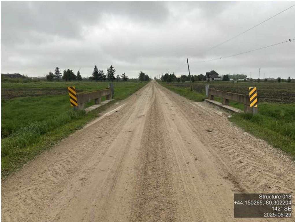
DECK WEARING SURFACE – SOUTHEAST
