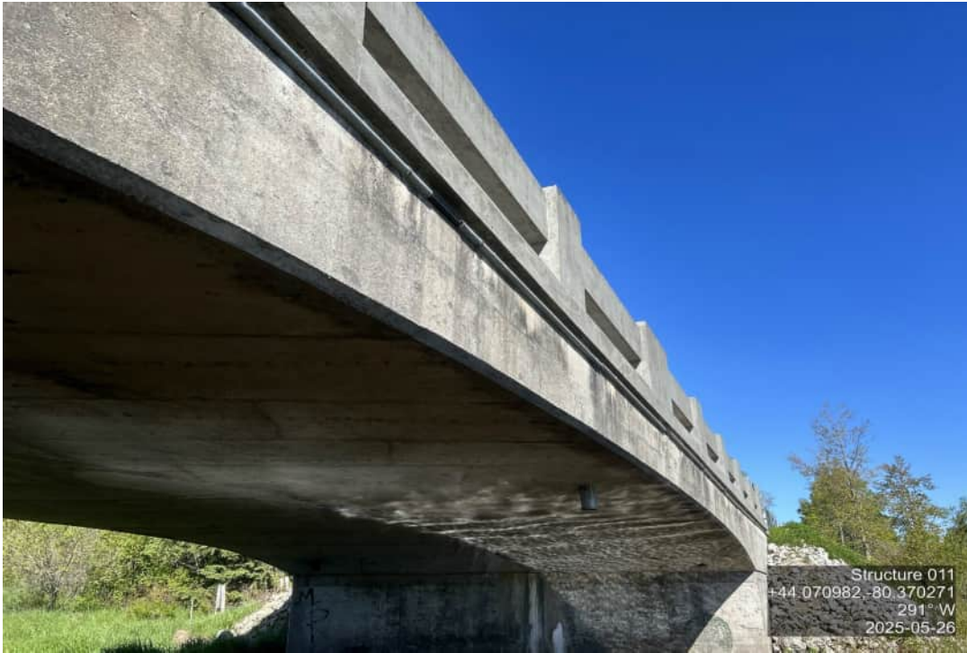
UTILITY – EAST – EXPOSED CONDUIT
