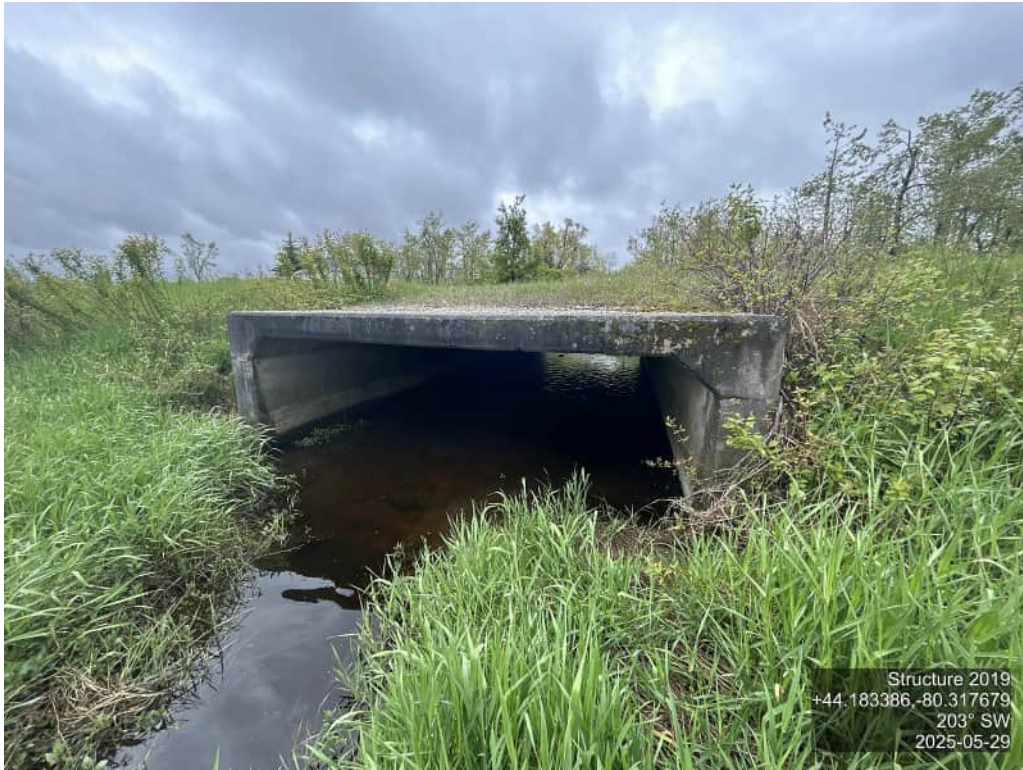
ELEVATION SHOT – NORTH
