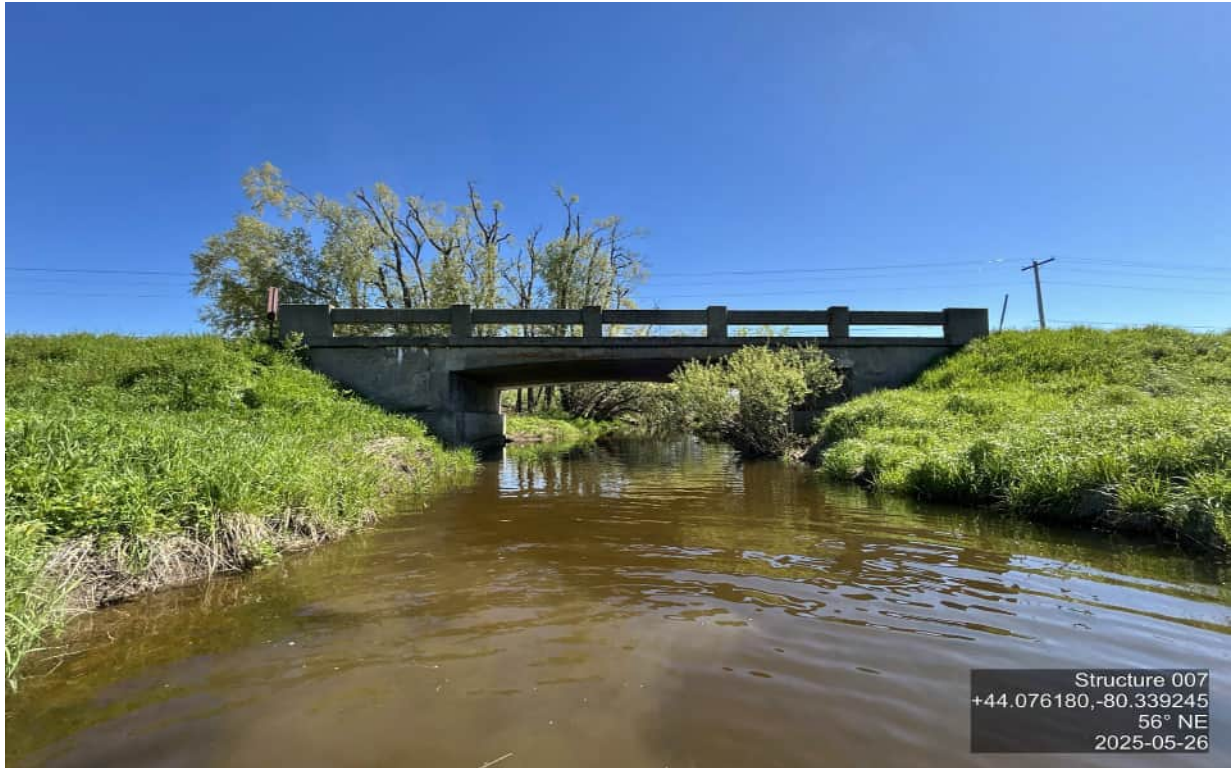
ELEVATION SHOT – NORTHEAST
