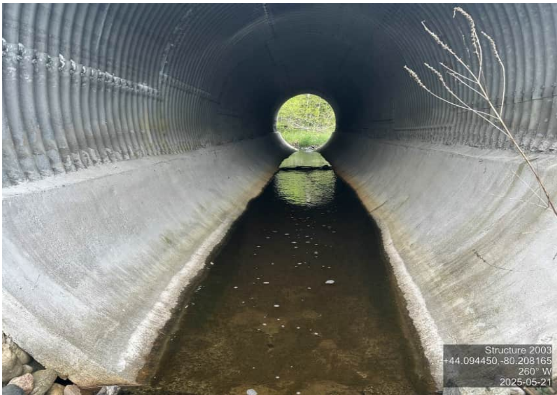
BARREL – WEST – SHOTCRETE INVERT PAVE (2019)
