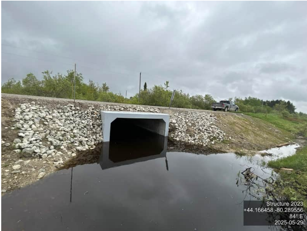
ELEVATION SHOT – EAST
