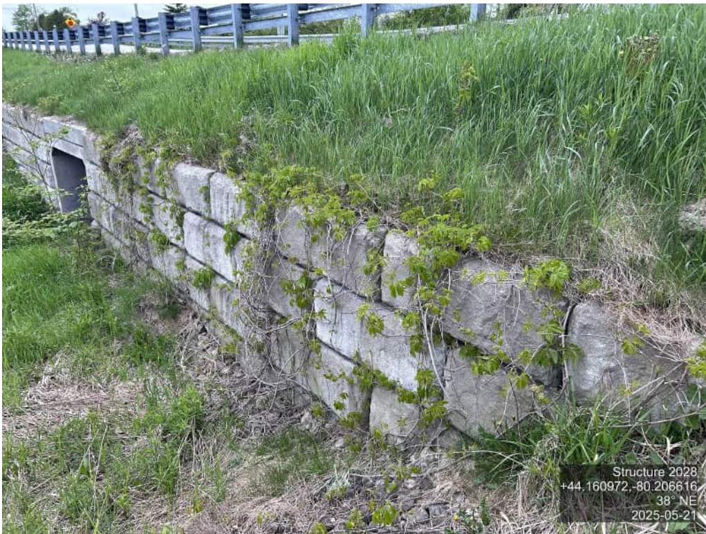
EMBANKMENT – NORTHEAST – ROCK PROTECTION
