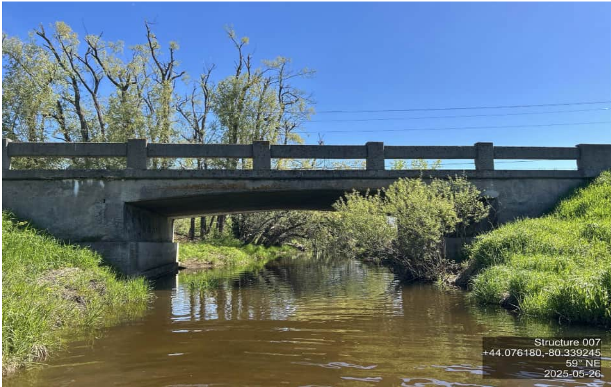
STREAM – TRHOUGH STRUCTURE – FLOWS WEST TO EAST
