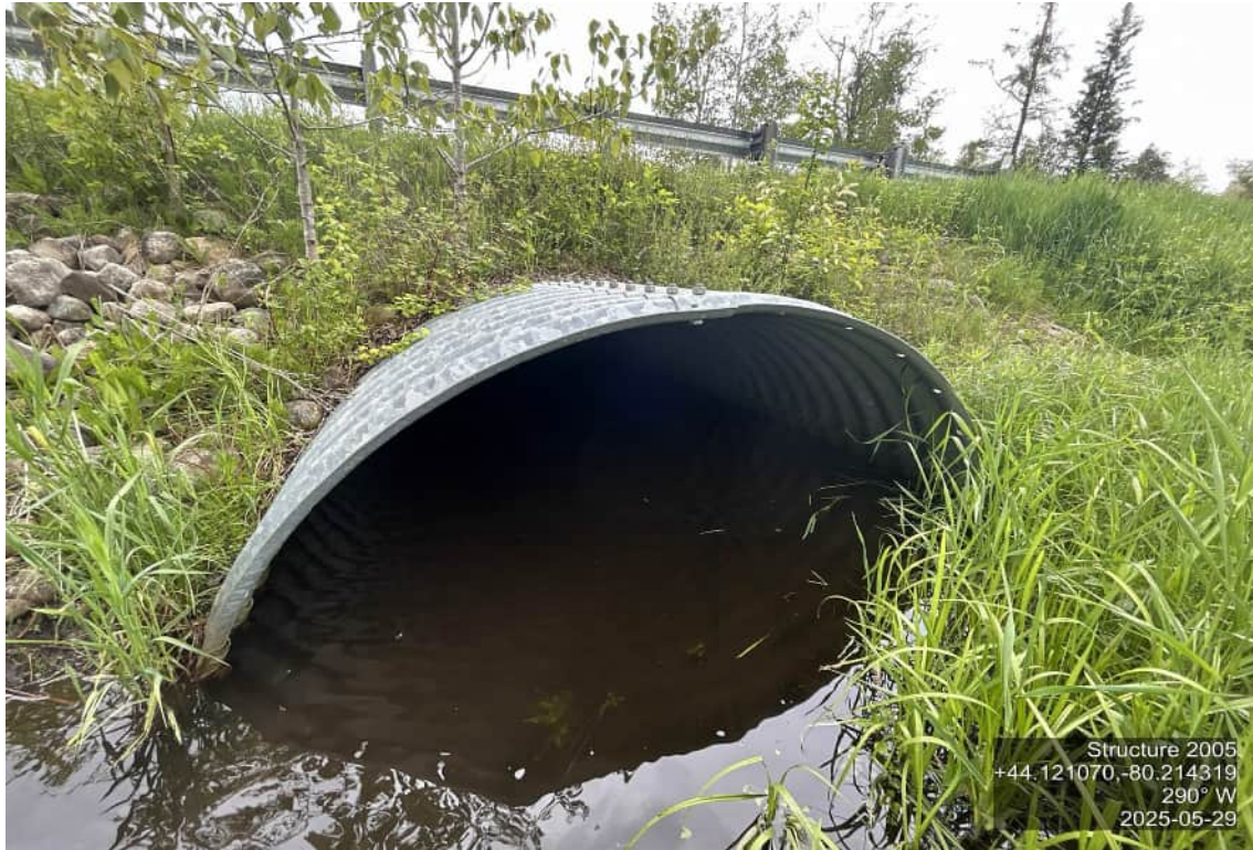
ELEVATION SHOT – WEST
