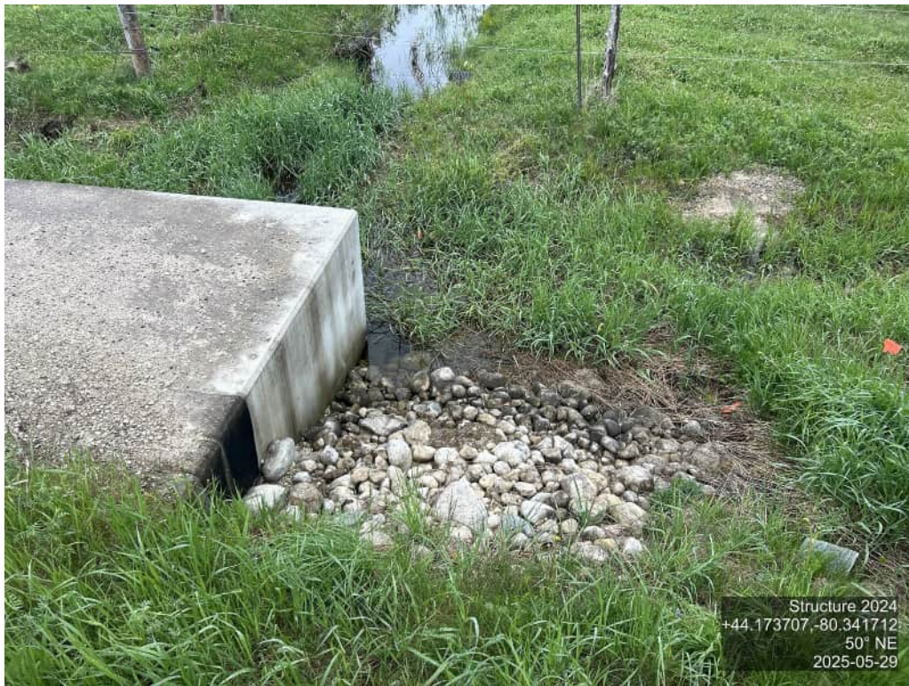
EMBANKMENT – NORTHEAST – ROCK PROTECTION
