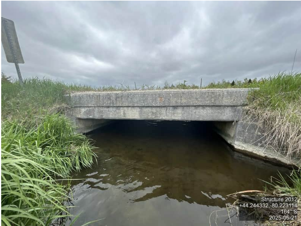
ELEVATION SHOT – SOUTH
