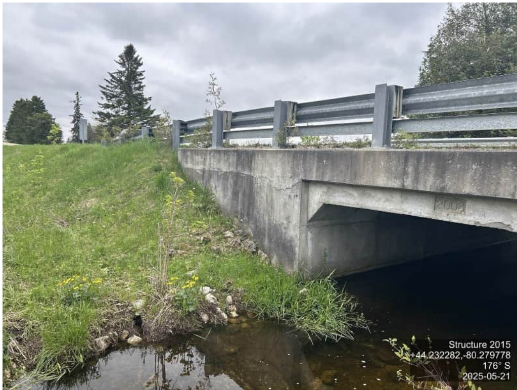
INLET – NORTH – SMALL GROUT REPAIRS PRESENT
