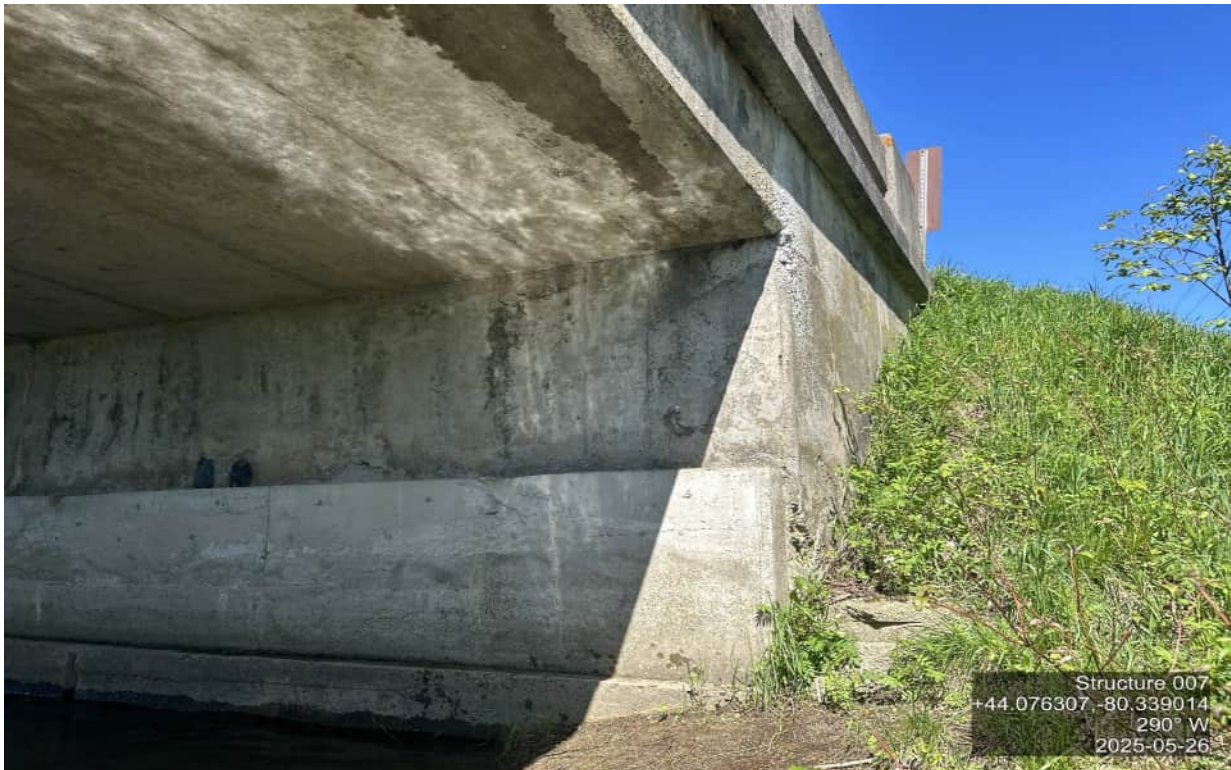
EMBANKMENTS – NORTHWEST – WELL VEGETATED AND STABLE
