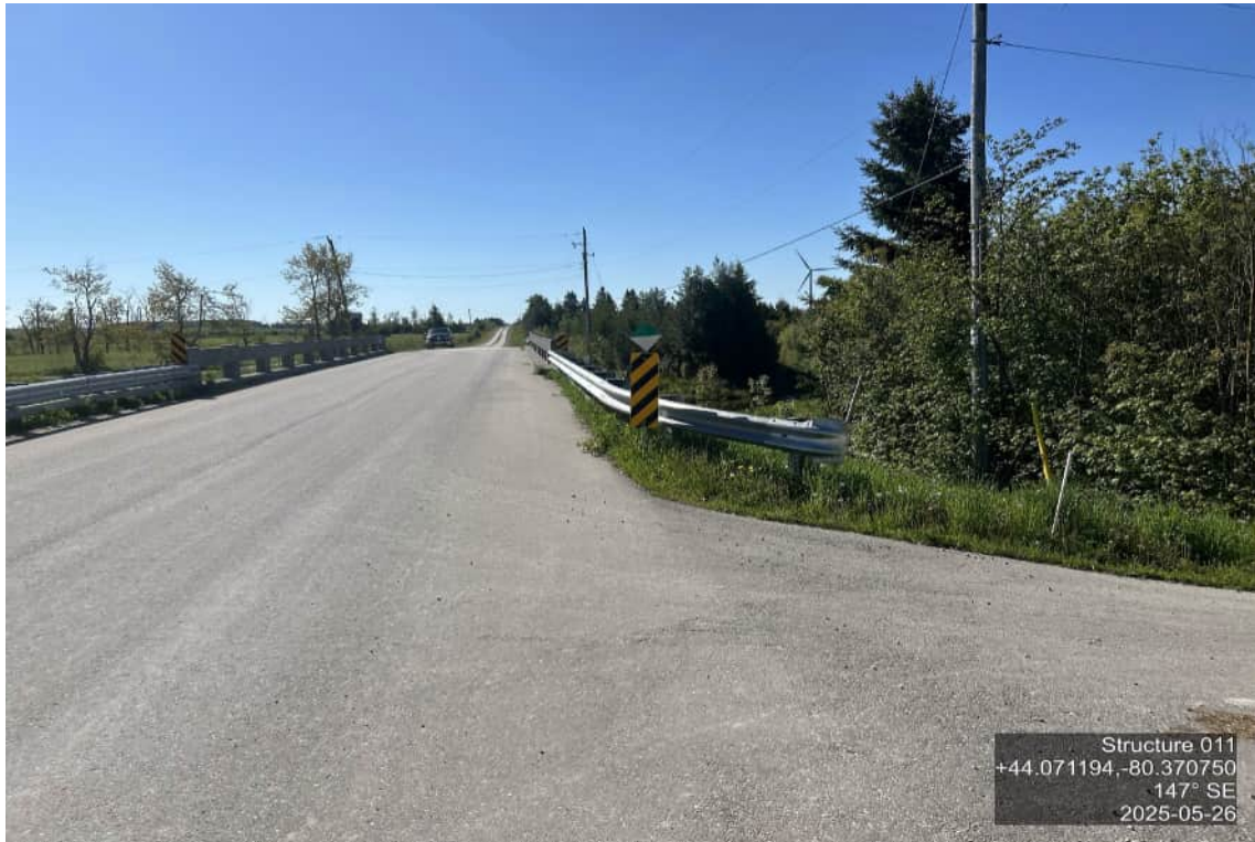
APPROACH GUIDERAIL – EAST – INSTALLED IN 2022 REHAB
