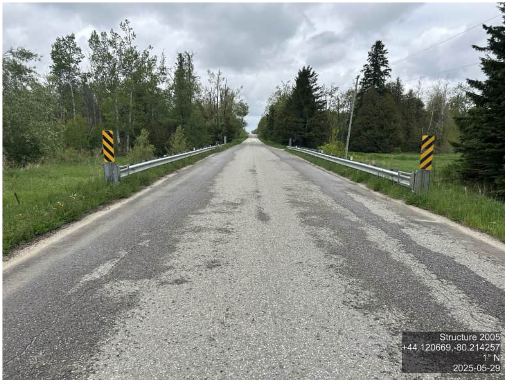
DECK WEARING SURFACE – NORTH
