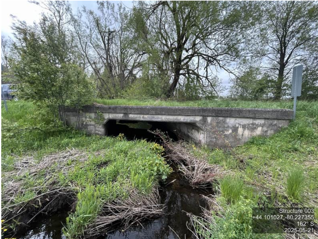
ELEVATION SHOT – NORTH
