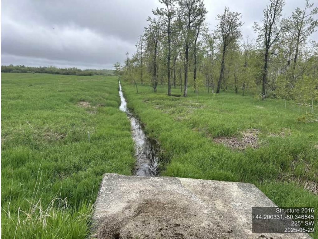
STREAM – WEST – FLOWS EAST TO WEST
